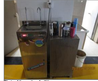
Photo of the sanitary facilities Drinking water.JPG
