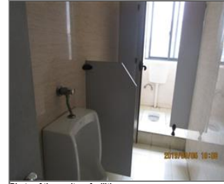
Photo of the sanitary facilities Toilet.JPG
